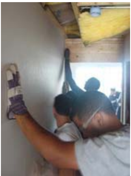
The team learns a new skill off the court - hanging drywall.
