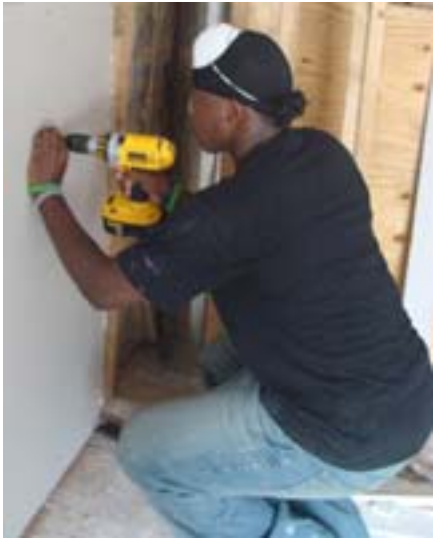
Preston Russell secures the drywall.
