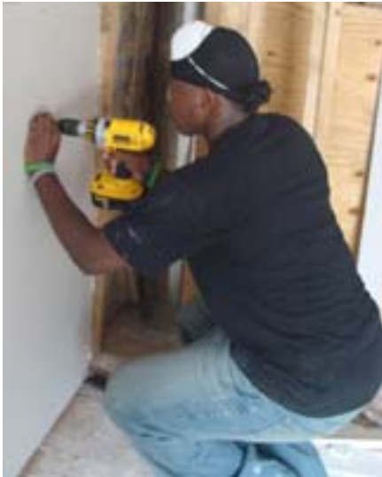
Preston Russell secures the drywall.
